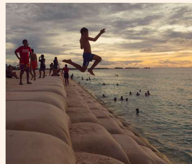
Liveti, 12, jumps from a sandbag staircase in Tuvalu that was built by the government to combat rising sea levels. The structure, called The Reclaimed Land, spans 78,000 m 2 – around 780 m long and 100 m wide – and is fortified on three sides with robust sandbags to hold back the ocean. ©UNICEF/UNI560974/Bak Mejivang
